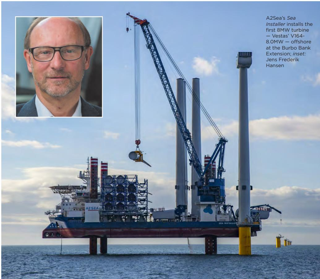
A2Sea's *Sea Installer* installs the first 8MW turbine — Vestas' V164-8.0MW — offshore at the Burbo Bank Extension; inset: Jens Frederik Hansen
